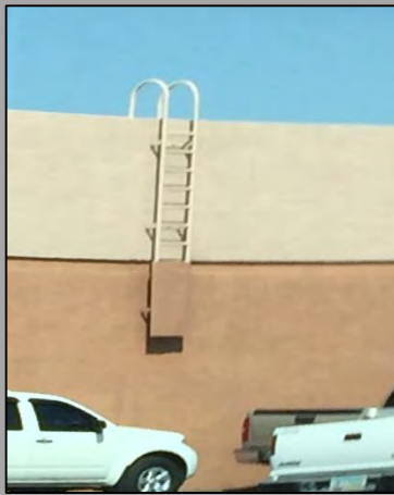
Ladder for building Roof Access
